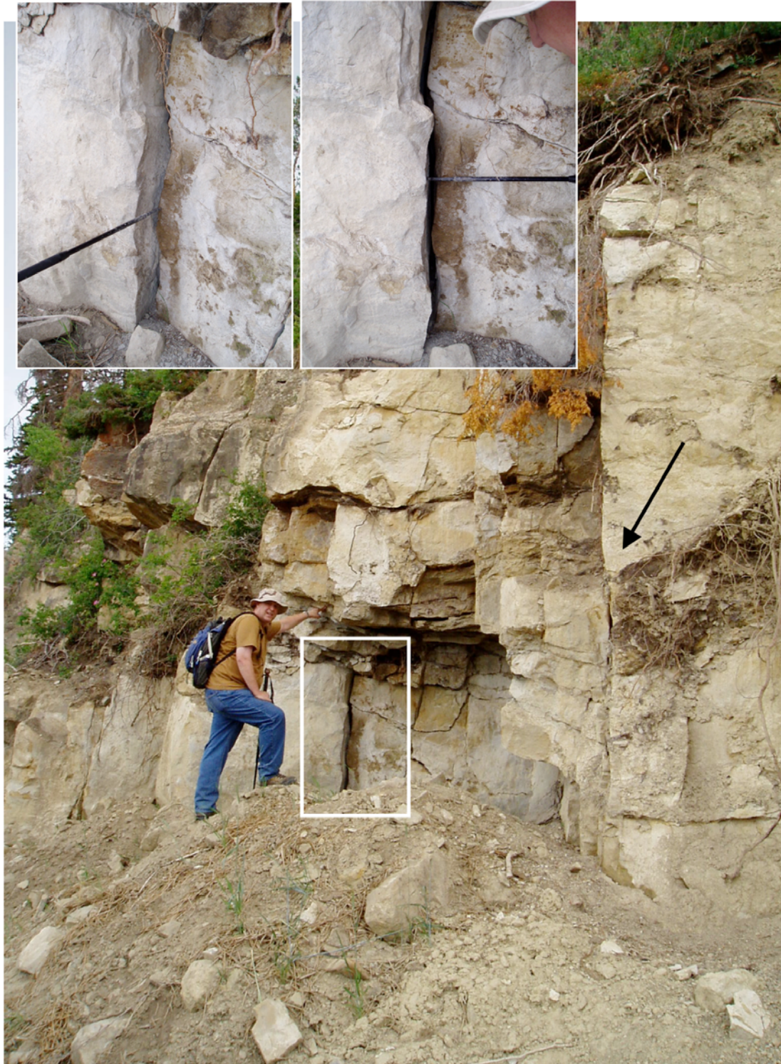
Figure 3.14. Massive fractured sandstone block at collapse site. Yellow line in Figure 3.13 shows location of this photo and strike of joints. Inset is blow-up of feature in white box. Arrow points to vertical joint with the discontinuous and apparently offset shaley unit. Author's advisor shown for scale.
